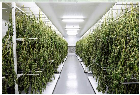
Darwin Chambers manufactures and installs drying rooms that can control temperature, air flow, additive humidity, and dehumidification at programmed (ramped) levels. This enables lot to lot consistency whether the drying happens in humid, coastal areas or dry, high altitude areas. Product can also be stored long term with precise levels of humidity to prevent mold or brittleness.
